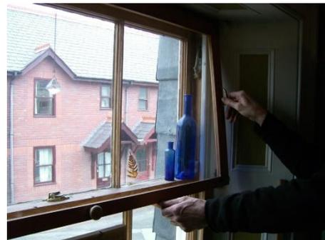
Hinged secondary glazing - bar aligned with original windows for a good match
